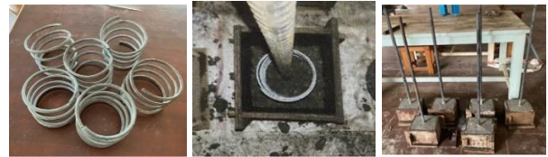
Fig. 4. Casting of pull out specimens
